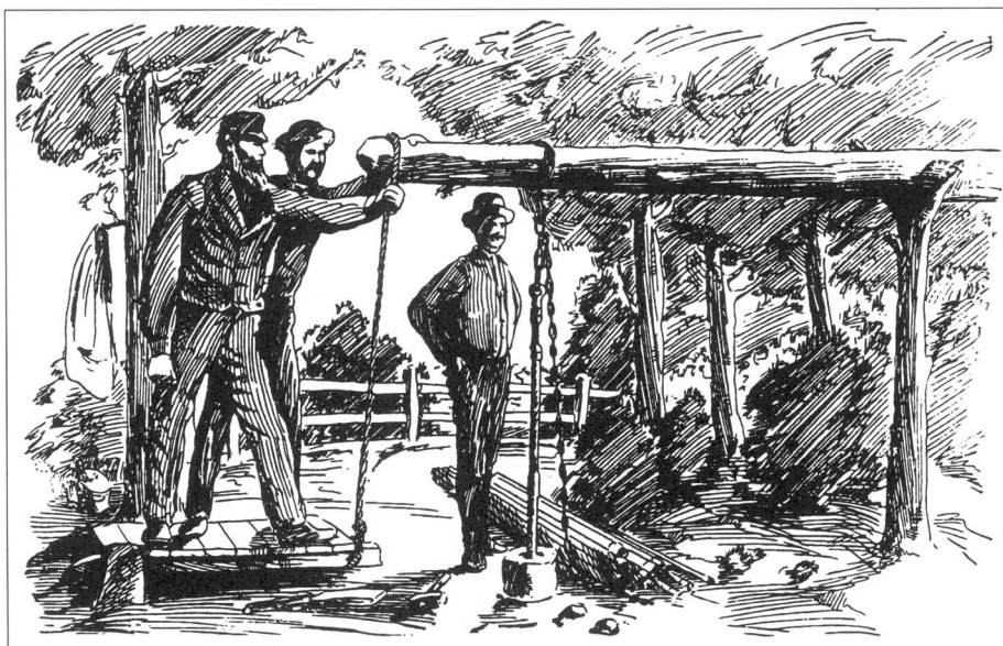
Figure 3: Spring-Pole Drilling Method
